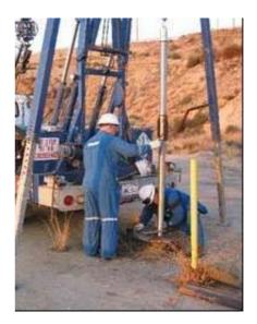
This flux tower being installed at a geologic storage site measures the concentration of gases in the atmosphere. Such devices can detect increases in  $CO_2$  Image source CO2CRC
